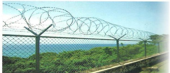
Chain link Fence
