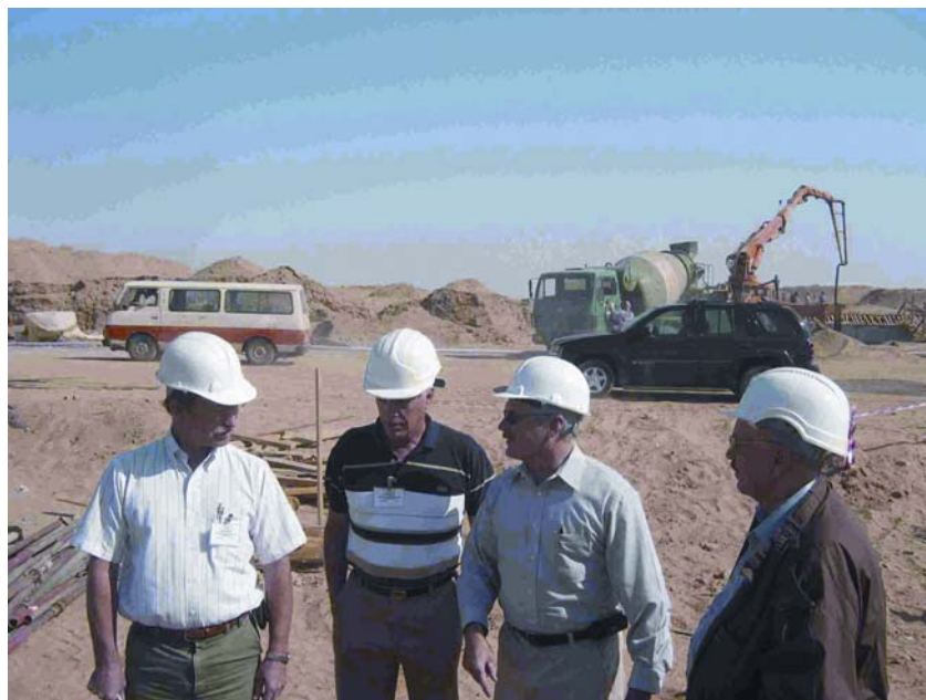
Critical human resources are also needed to address strategic priorities such as those in the Middle East. In this photo, the USAID/Jordan Water Resources Office Director James Franckiewicz reviews the progress of work at the Aqaba Wastewater Treatment Plant.
