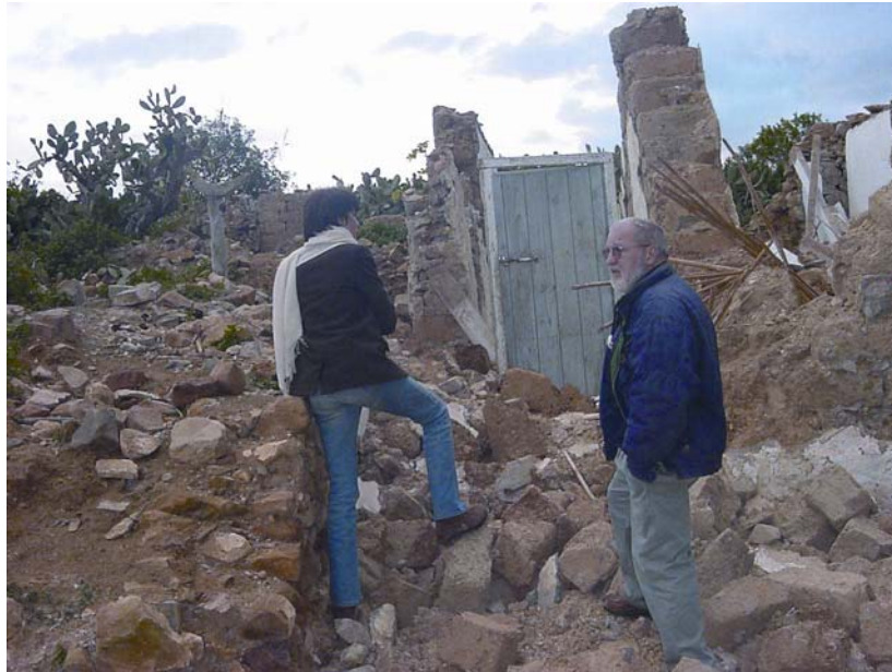
Former USAID/Morocco Director Jim Bednar (now mission director in Zambia) and DART team member Regina Davis assess earthquake damage in Al Hoceima in February 2004.
